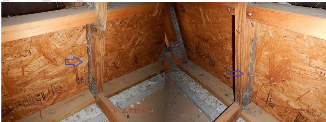
**Type of Roof to Wall Connectors:** Standard Metal Straps/ Good condition at accessible areas of the Attic
