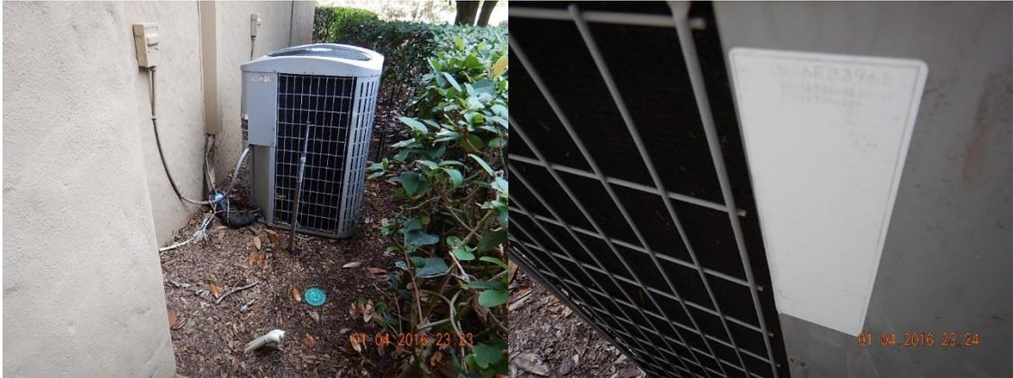
Two of the Condenser Units are installed at the north side of the building/ These are for the Master Bedroom and the First Floor Main Living Area Systems
