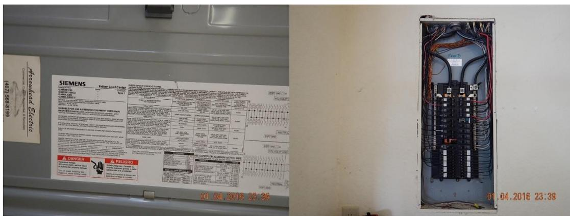
**Sub Panel B Location:** West Interior Garage Wall- Visible and accessible wiring appeared to be in good condition at the time of the Home Inspection
