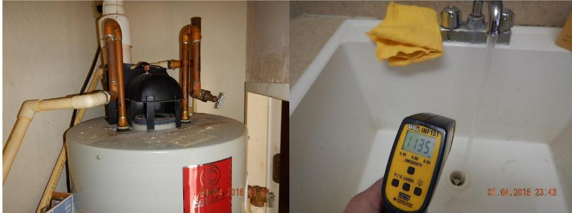
Infrared Thermometer was used to verify the Water Heater was producing hot water at the time of the Home Inspection
