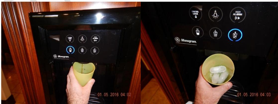
Kitchen- The Ice Dispenser for the Kitchen Refrigerator is not fully functional/ The Ice gets stuck and jams up when using the Dispenser
