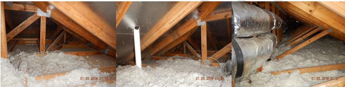
**Attic Insulation:** R- 30 Loose Fill Fiberglass-Fiberglass Batt-Radiant Heat Barrier/Good condition and evenly installed throughout accessible areas of the Attic
