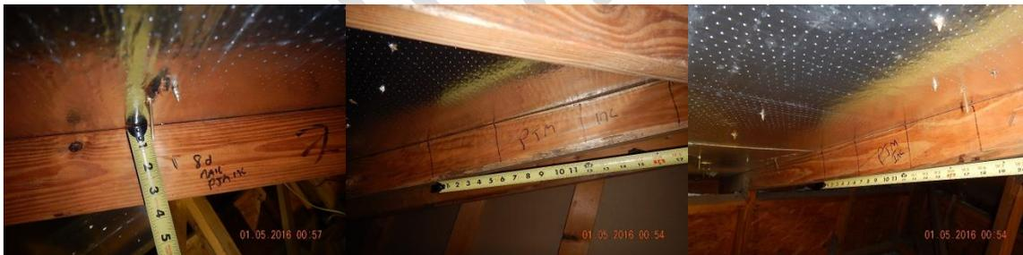
**Roof Decking Attachment Nail Size & Spacing:** 8d nails spaced a maximum of 6" apart in the field/ I used a Metal Detector to locate and estimate the nails and calculate the spacing
