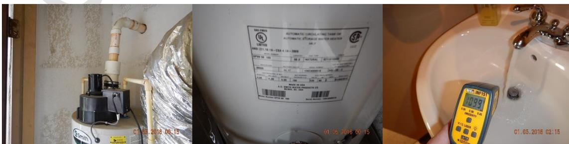
The Water Heater at the Second Floor West Balcony Closet appeared functional and in good condition/ The Water Heater was replaced in 2012 and produced hot water during the Home Inspection
