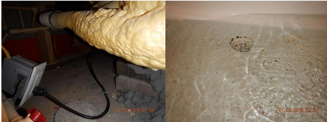
There is dirt in the Tub Jet System and the Air Blower function appears compromised at this time/ The Service Access Panel is installed the left side of the Tub/ GFCI Protection was verified
