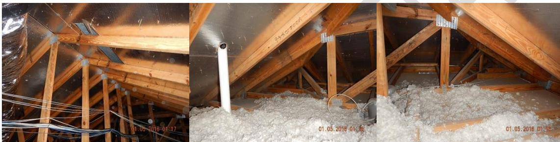
**Type of sheathing:** 15/32" Plywood/ **Condition:** Good condition at visible & accessible materials- Radiant Heat Barrier inhibited viewing access to the majority of the Roof Deck Materials
